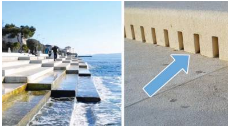
Figure 8: Staircase in Zadar.
